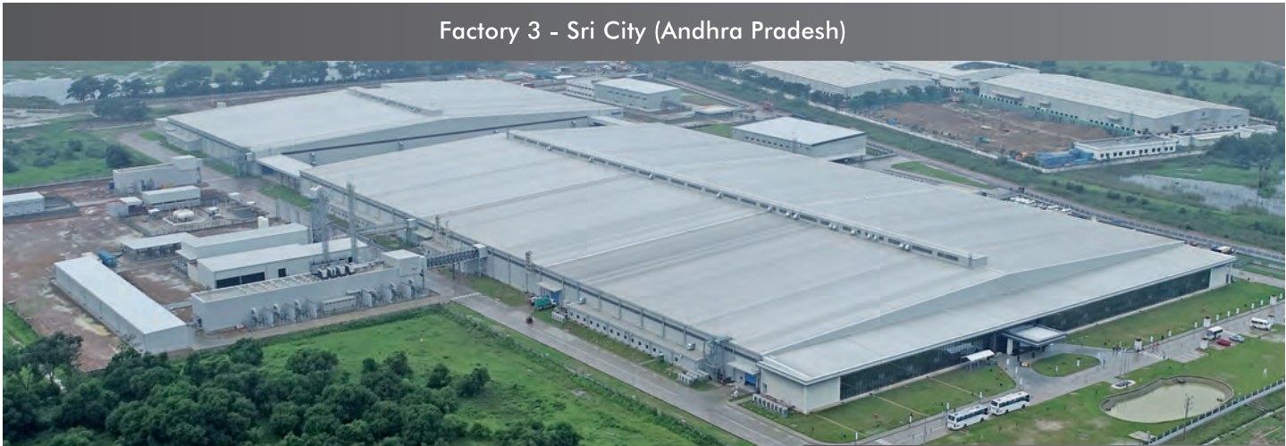
Compressor & Device manufacturing facility
