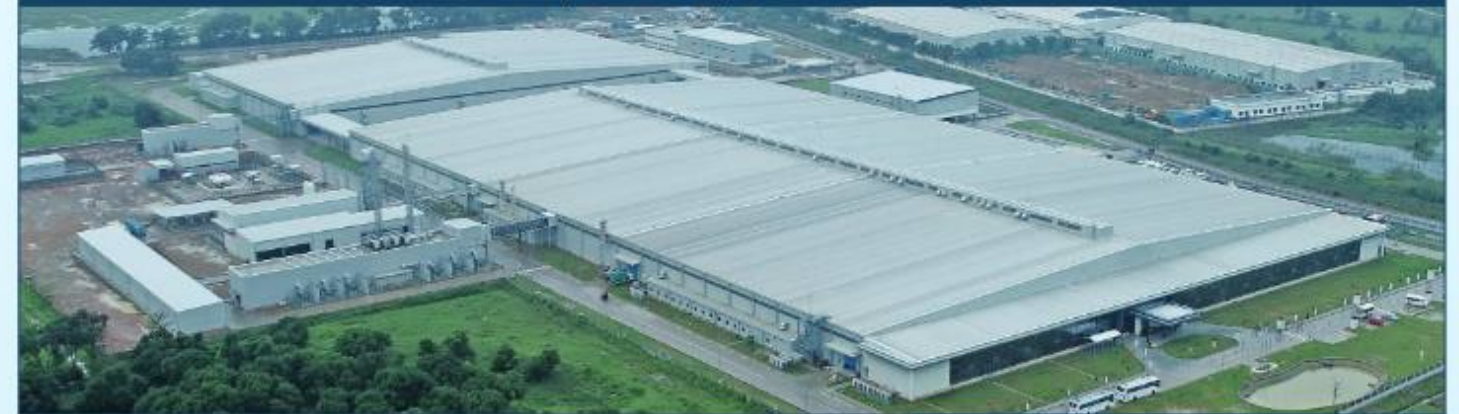
Compressor & Device manufacturing facility
